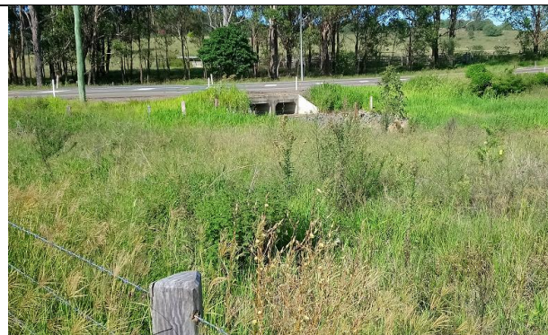
Photograph 2 – Culvert discharging into channel north of the Project area.
