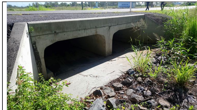
Photograph 1 – Existing box culvert
