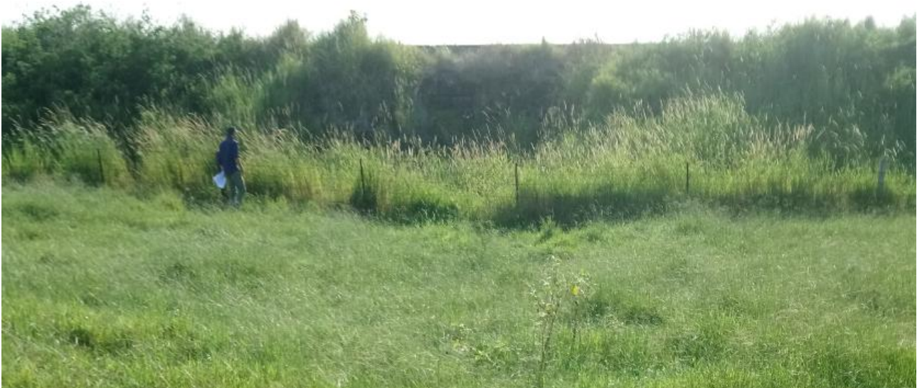
Photograph 4 – View of culvert passing under railway line.
