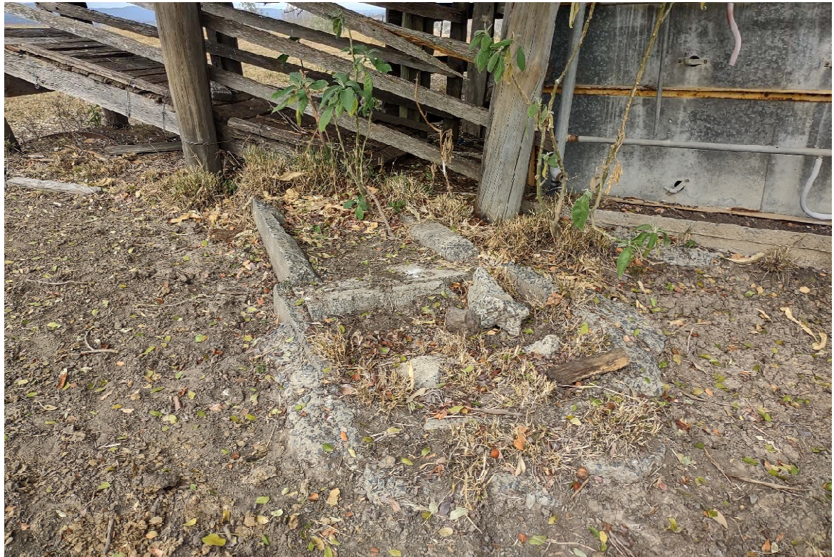
Photograph 9: View of concrete slab
