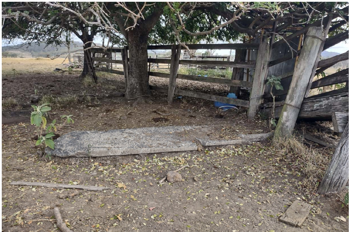
Photograph 10: View of concrete slab
