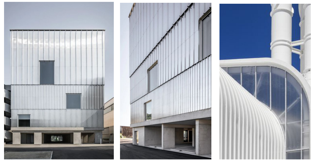
Metal cladding with vertical element at varied spacing across bands
