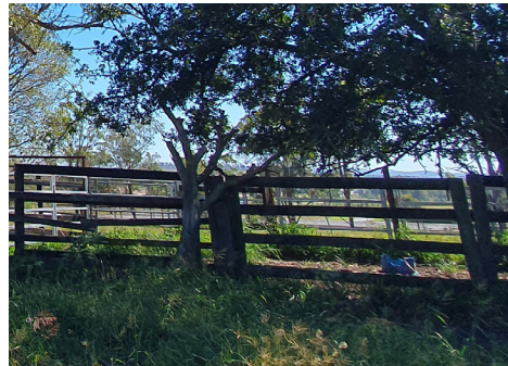
Existing farm fence structure
