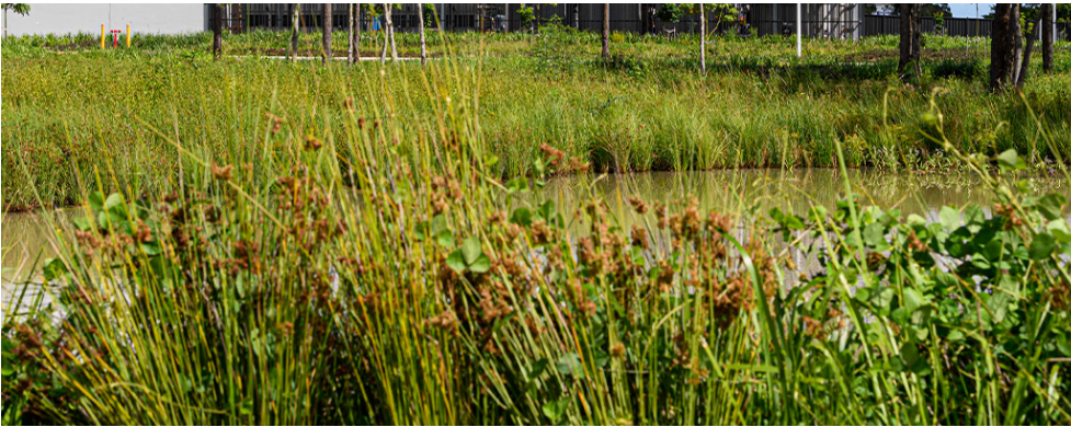
Vegetated stormwater basin
