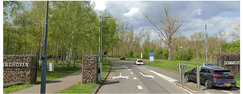
Feature entry gate and signage
