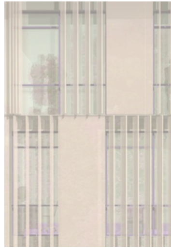
Perforated metal panels and louvres
