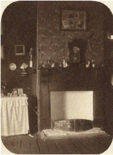
Figure 4 Interior view showing a bedroom at Bromelton Station (2007. Interior view showing a bedroom at Bromelton Station, John Oxley Library, State Library of Queensland).
