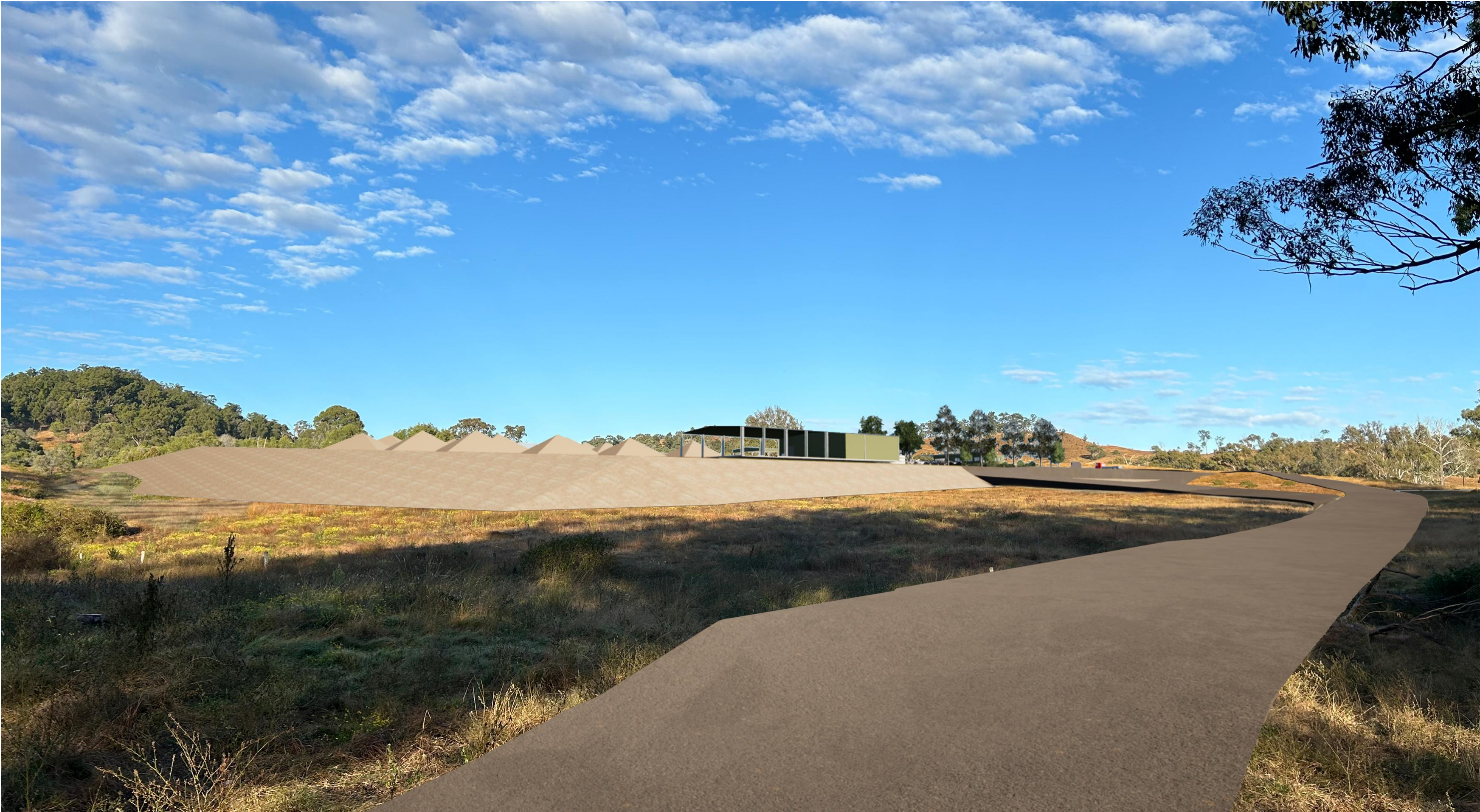
1 Site View from Mitchell Road
