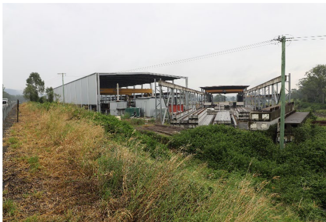
Photo 5 An industrial site along Beaudesert – Boonah Road
