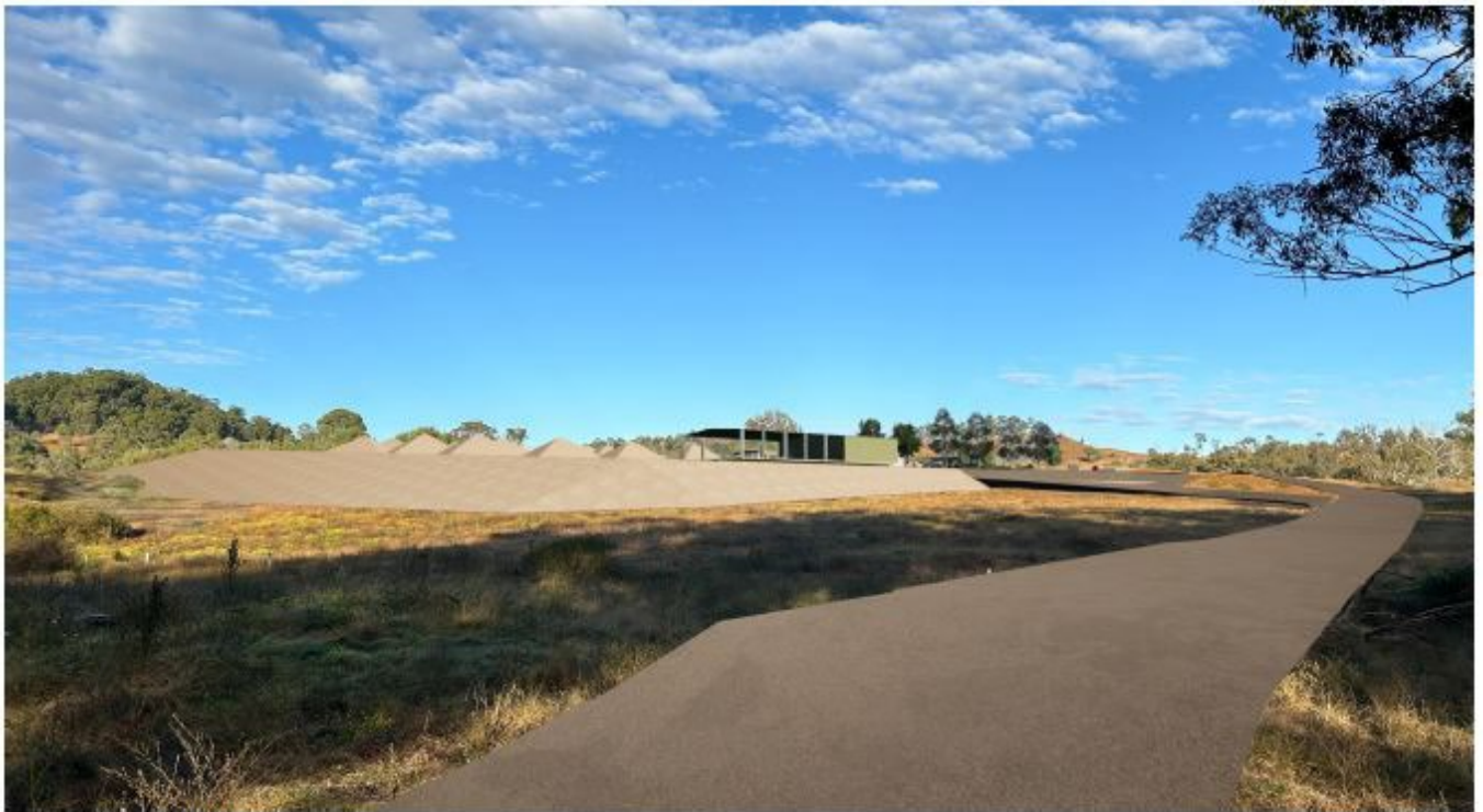
1 Site View from Mitchell Road
